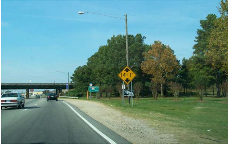
Existing entrance adjacent I-95
