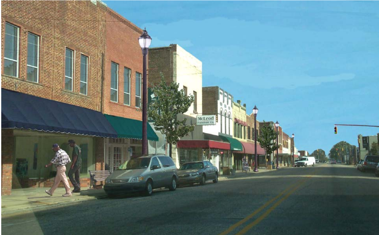
Downtown After - with restored facades, windows, new lighting, underground utilities and street trees.
